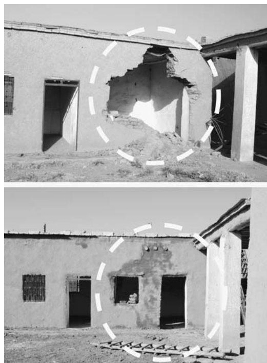
Figure 3. A HOLE IN THE WALL OVERHAULED: Damage to the dig house following winter rain and vandalism: (above) collapsed doorway and window in northwest corner of inner courtyard, the residential quarter of the dig house (October 2004); (below) doorway following repair of walls and roof (April 2005)
