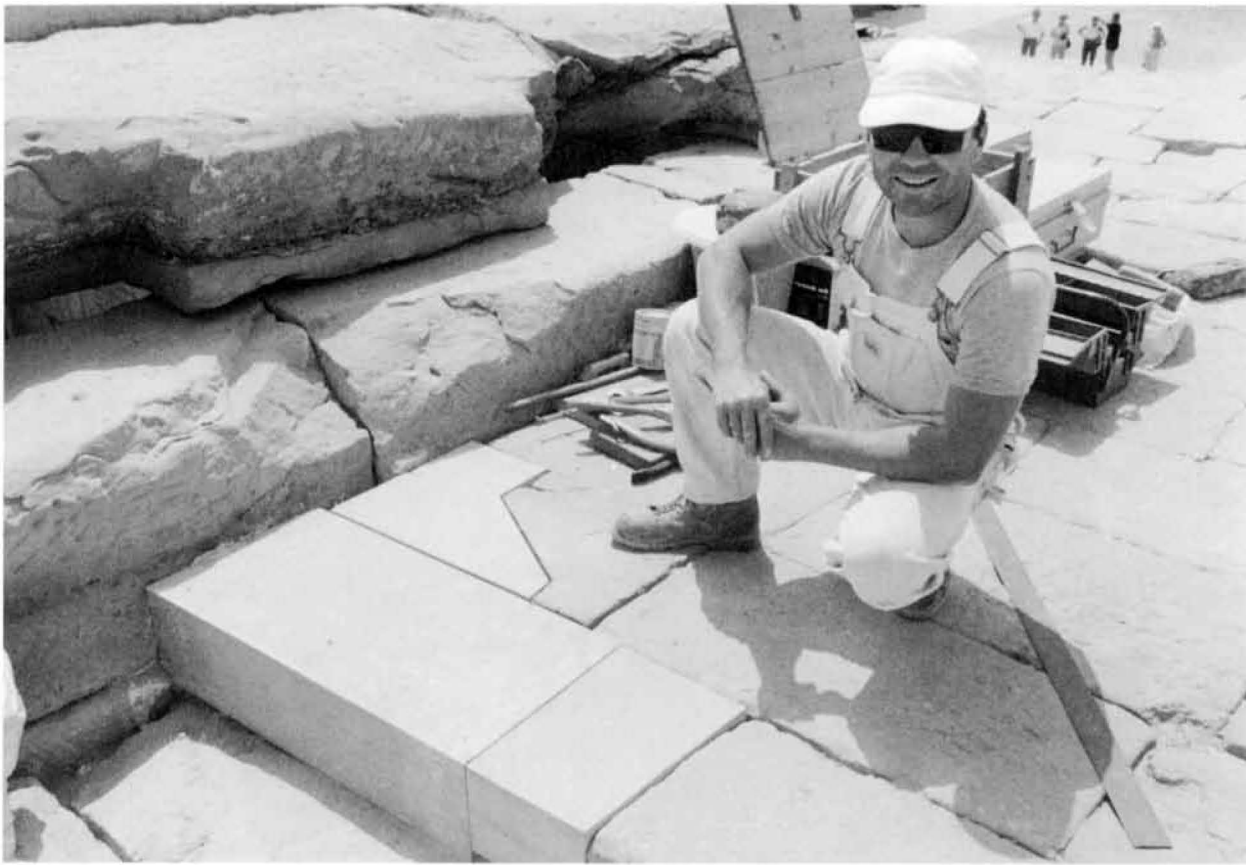
Stonecutter Dany Roy with newly restored sandstone roofing blocks, Eighteenth Dynasty Amun temple roof, Medinet Habu, March 2000. Photograph by Ray Johnson
