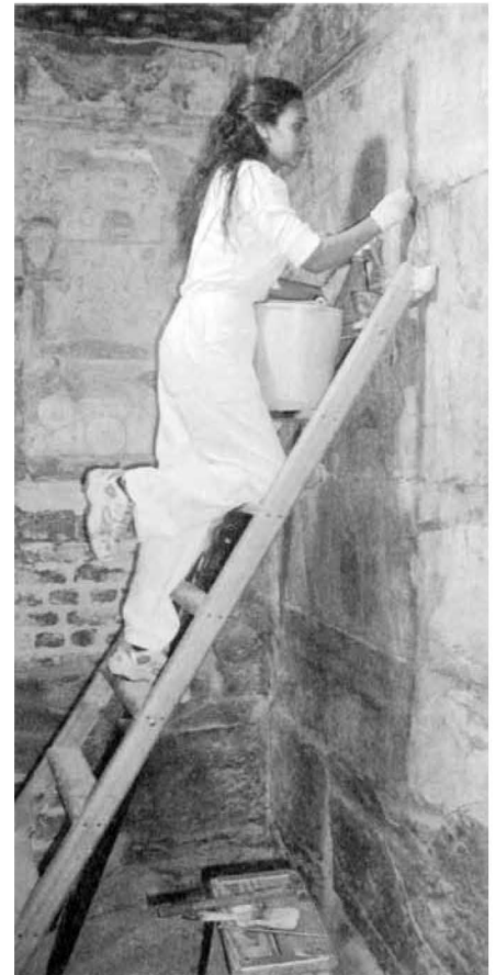
Nahed infilling gaps in the wall, naos room, Medinet Habu
