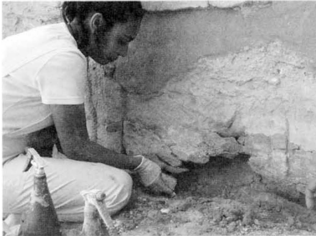
Nahed consolidating Ptolemaic wall, MHB.
