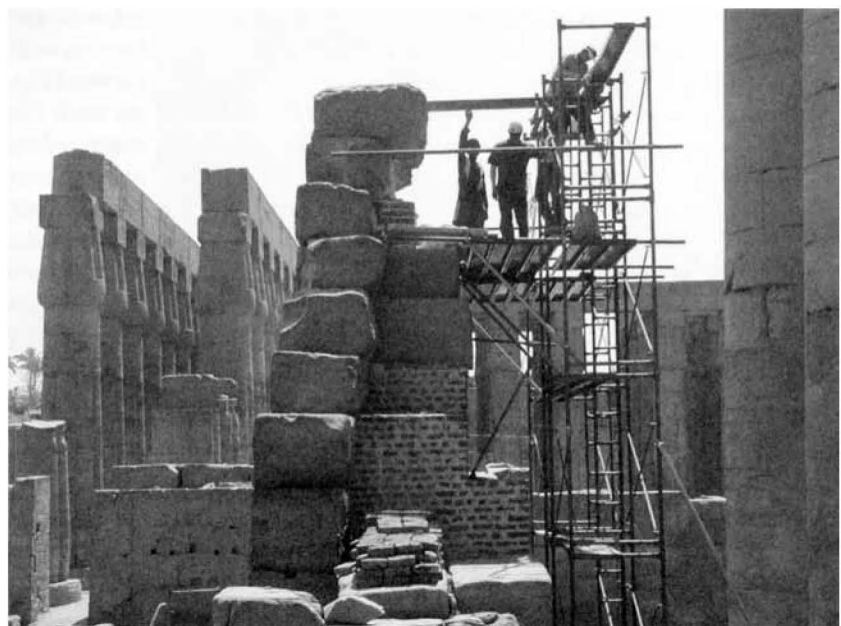
Brick buttress from north, eastern wall, Colonnade Hall.
