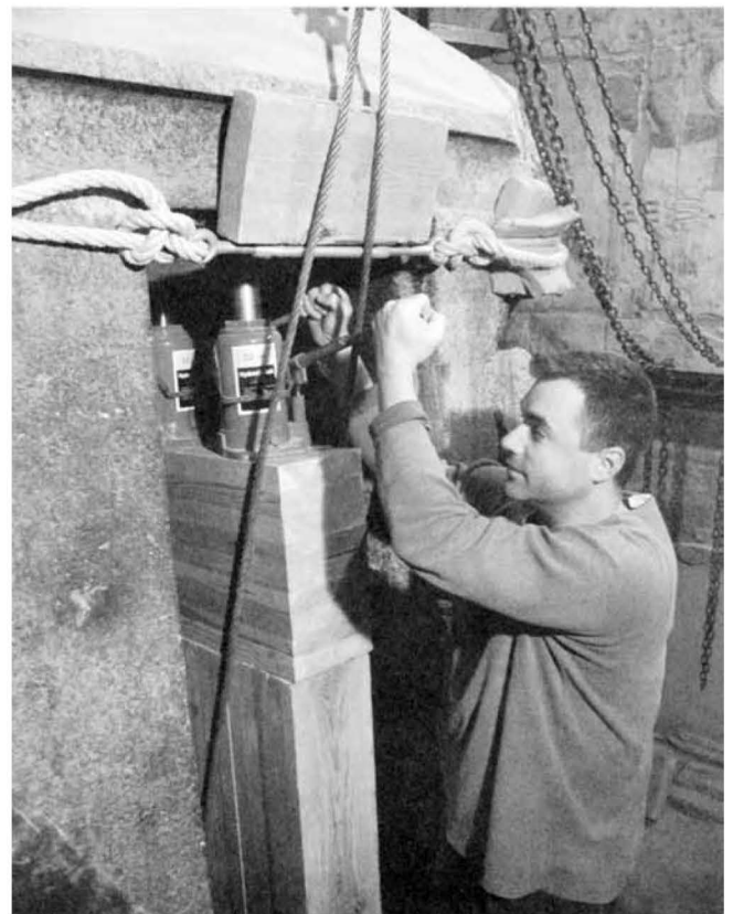
Dany jacking granite naos into position for restoration and moving, MHB.
