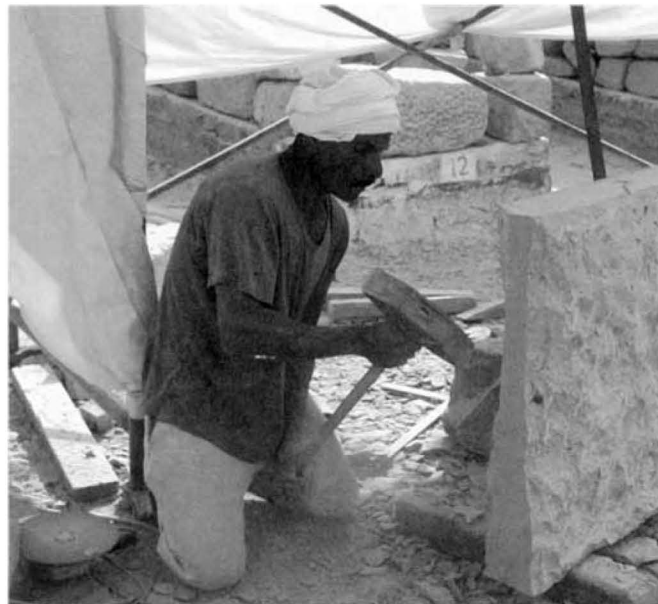
Stone cutter Gamal shaping a veneer stone, Luxor Temple blockyard.
