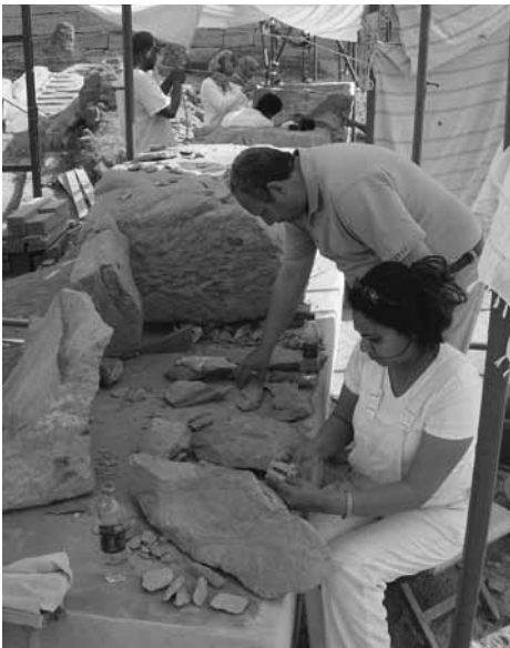
Adel, Nahed, and conservation team consolidating well blocks at Medinet Habu
