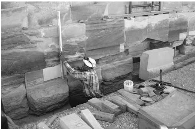
Ali patching sanctuary wall at Medinet Habu
