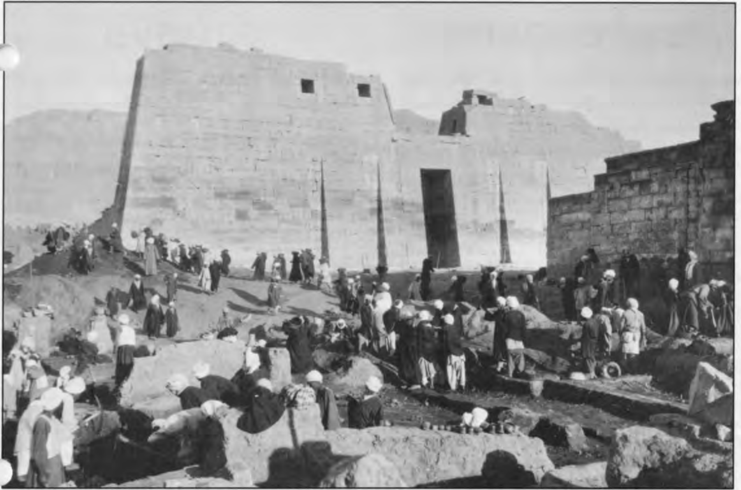
View of the work in the southeastern section of Medinet Habu about 1929
