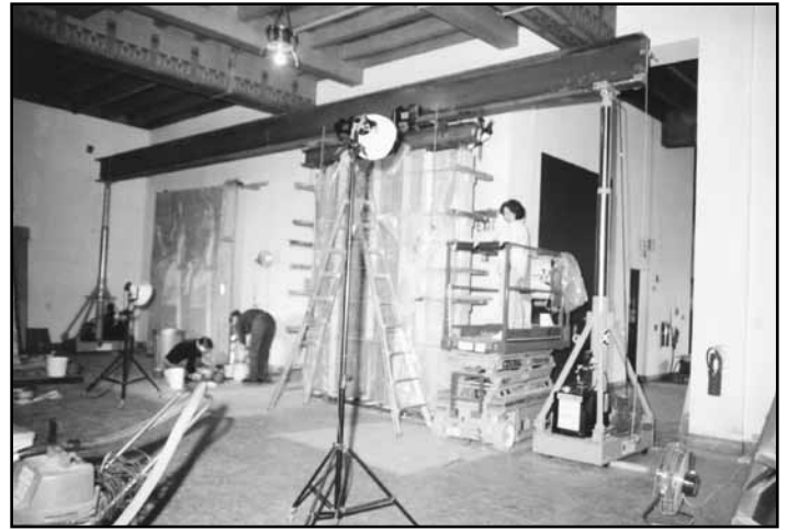
First two reliefs in Khorsabad Court being installed by Laura D'Alessandro, Vicky Parry, and Vanessa Muros
