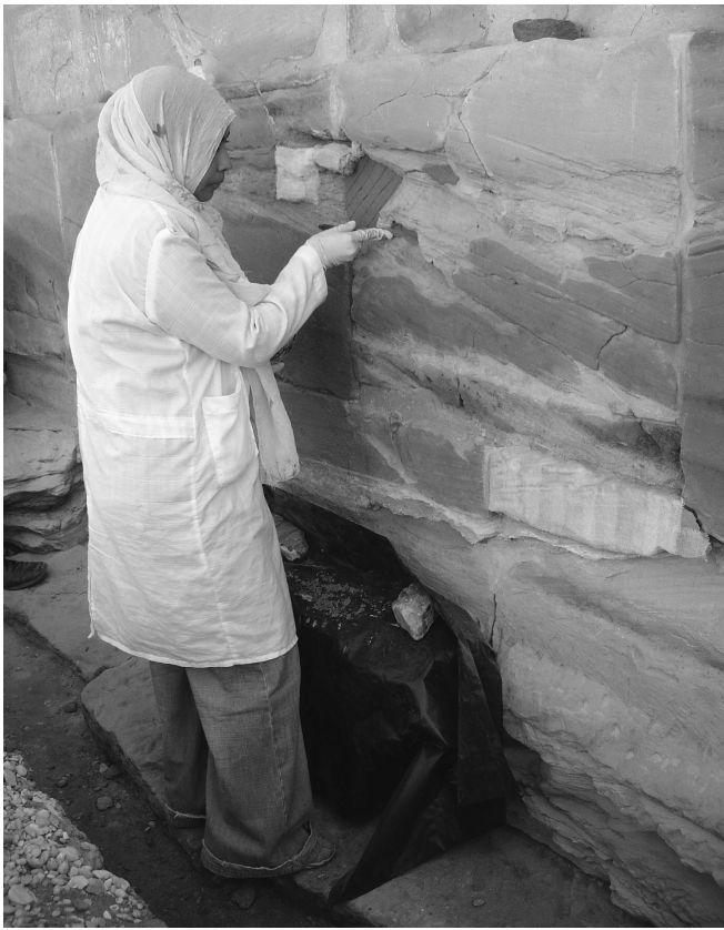
Conservator Hala consolidating the back wall of the small Amun temple sanctuary
