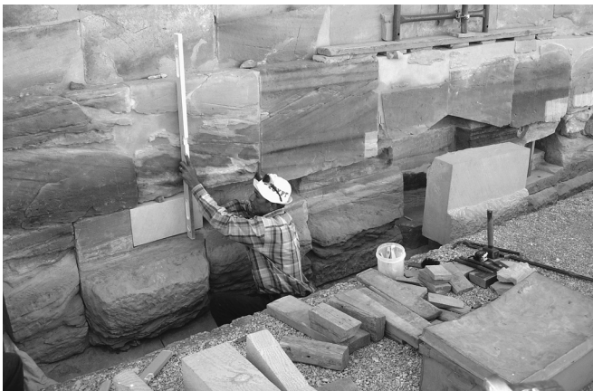
Ali patching sanctuary wall at Medinet Habu
