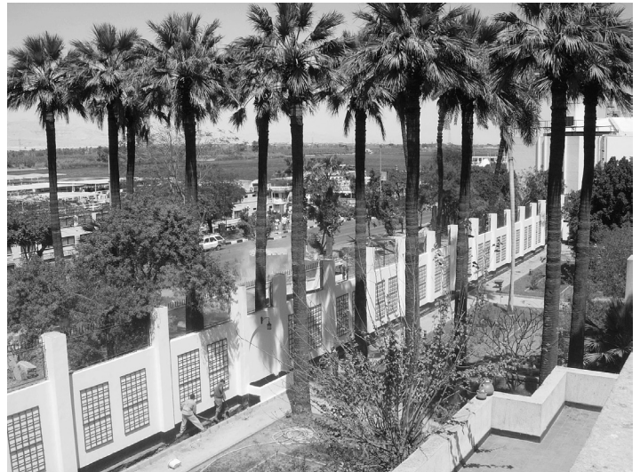
The completed wall from above
