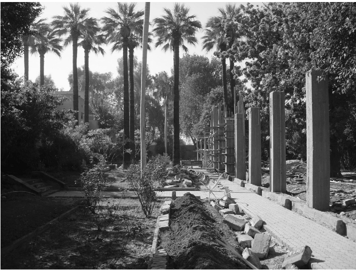
Chicago House garden, new wall going up, December 12, 2008
