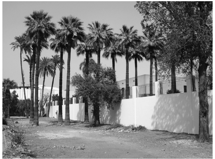
The completed wall from outside
