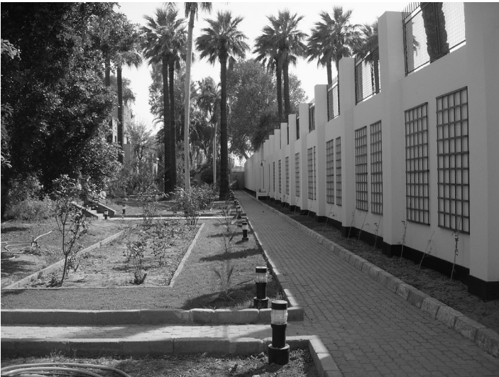
The completed wall from inside
