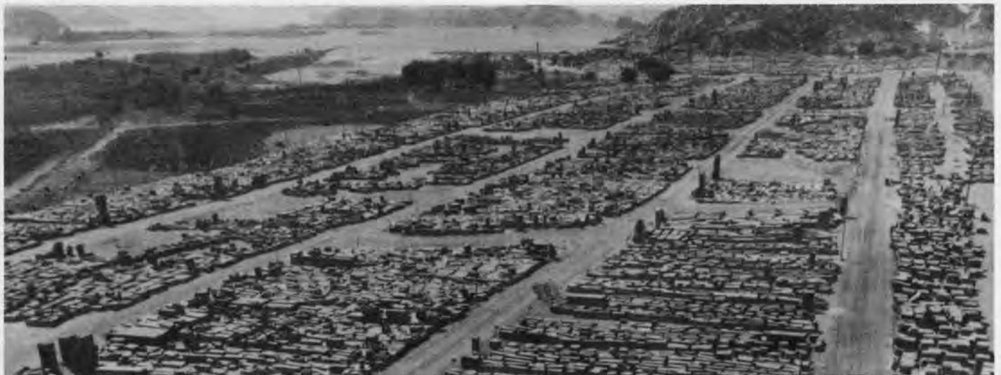
37,363 separate blocks were shipped to the bank and kept in storage while Agilkia was made ready to receive them.
