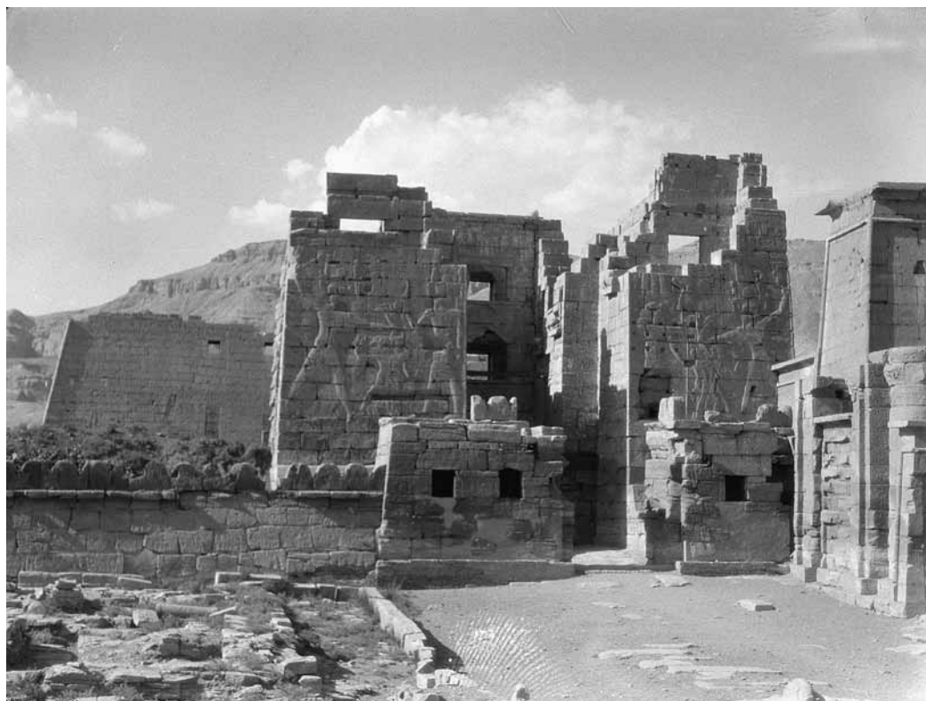
FIGURE C14.1. The facade of the Temple of Ramesses III at Medinet Habu showing the condition of the walls and gate in 1931 (Oriental Institute field negative E1/O46)
